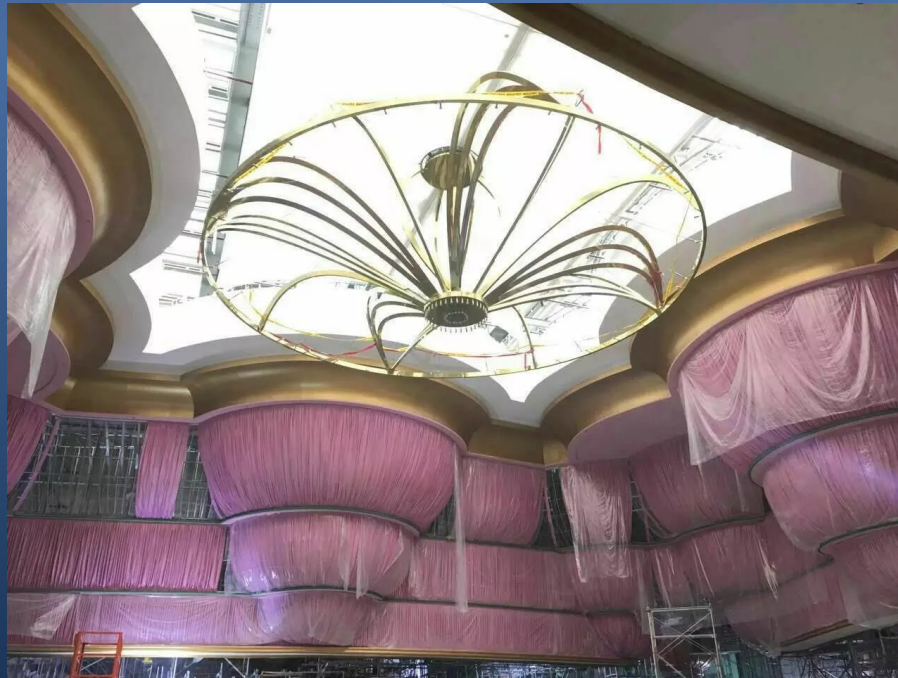
GRP Column Features Semi-Product Assembly
